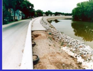
Ft. Wayne Indiana Floodwall
