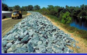
American River Levee
