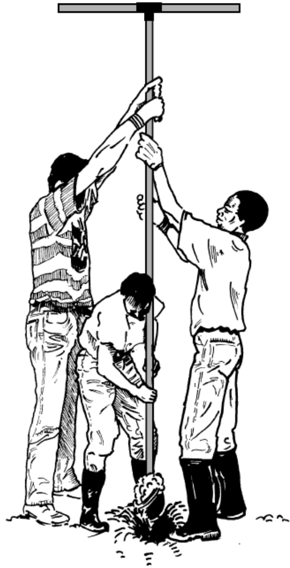
Hand-auger drilling for boreholes up to 10m deep
